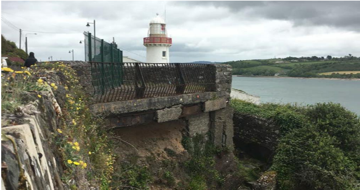
Lighthouse Viewing Platform
